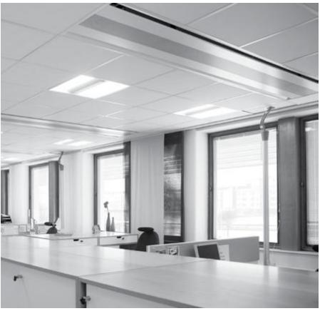
Figure 36: Krueger Chilled Beam Office Application.
